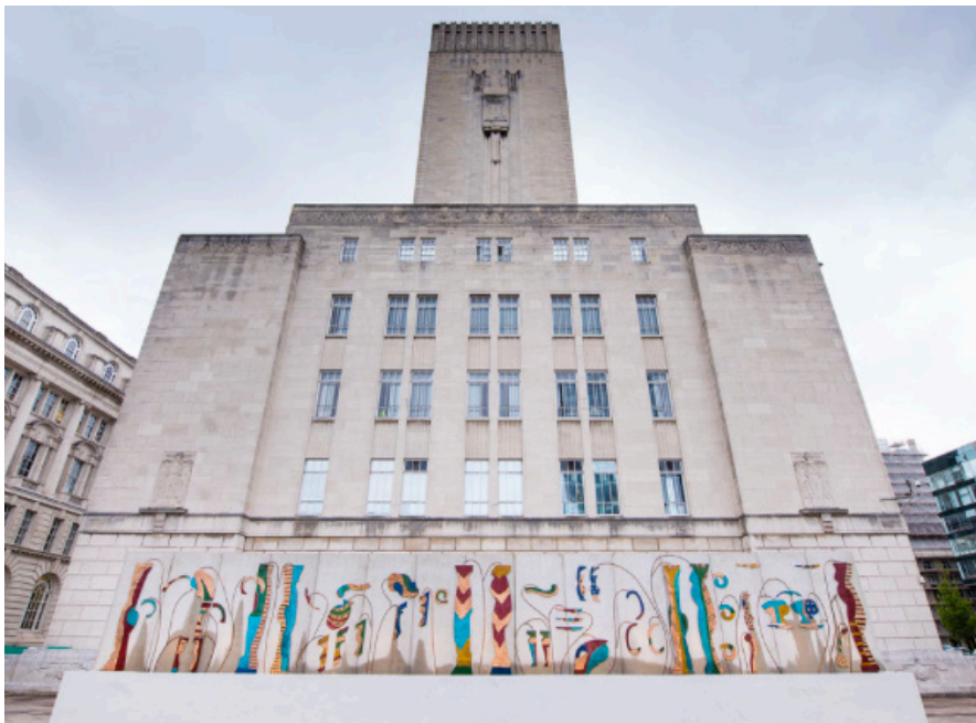
Betty Woodman. Liverpool Fountain , 2016. Bronze, patina, copper piping. 15 meters long. Commission for Liverpool Biennial 2016. Installation view at George's Dock Ventilation Tower Plaza, Liverpool, England. Photo by Joel Chester Fildes.
