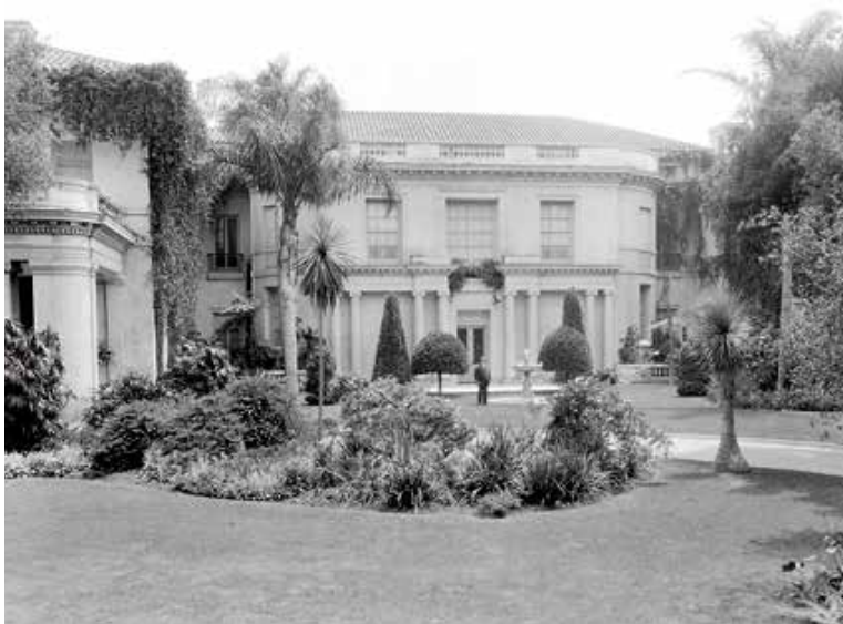
Fig. 2 Henry E. Huntington standing in front of the north façade of the Huntington residence, circa 1915. Reproduced by permission of the Huntington Library, San Marino, CA
